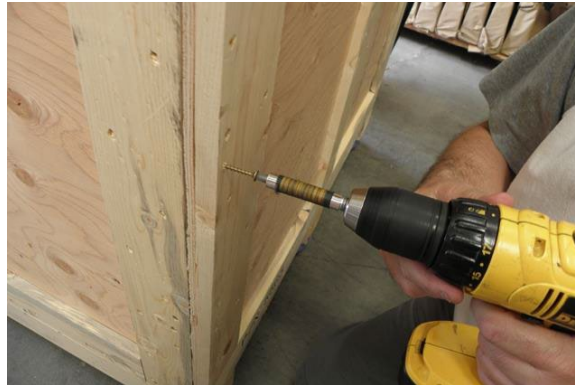
Figure 1. Removing Screws from the Shipping Container
